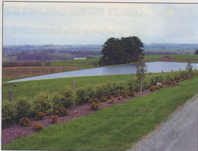
Dream-time Wholesale Nursery collects rainwater and run-off in its 80-million-litre dam.
